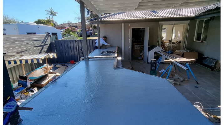
Composite Deck & Pergola – Long Jetty
