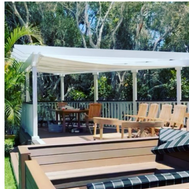
Structural Bifold Door Installation
